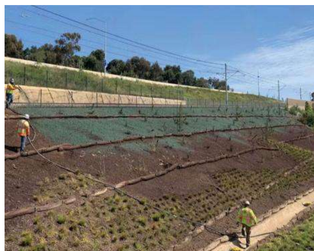
Figure 1 Hydroseeding in action. (Source: https://krishijagran.com/agripedia/how-hydroseeding-helps-farmers-in-preventing-soil-erosion-and-grow-lush-healthy-pastures/ )
