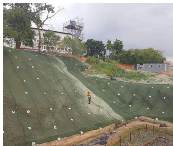
Figure 3 Maccaferri's MacMat installed on top of hydroseeding to reinforce a riverbank so it can withstand fast-flowing currents. (Source: https://dialogue.earth/en/climate/4-innovations-that-can-be-part-of-india-bangladeshs-flood-defences/ )
